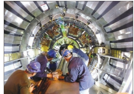
Technicians work to install the central section of the beam pipe, part of the CMS experiment.
